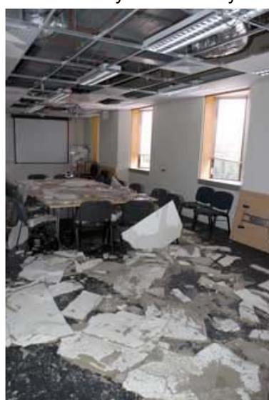
APSR is housed in the Hancock Library on the ANU campus, and the offices suffered water damage (as seen in image above). The gutters were blocked by hail so rain seeped in to the ceiling, dripping onto computers and desks.
